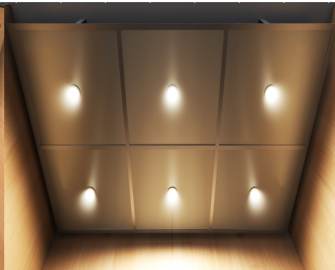
Drop ceiling with brushed aluminium panels and downlights
